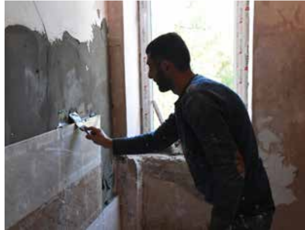
Kindergarten N 1 under renovation
